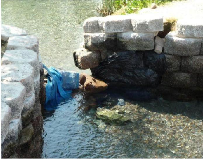
Figure 2. Ash Springs pool, large portions separating from the rest of the wall. June 6, 2013.
